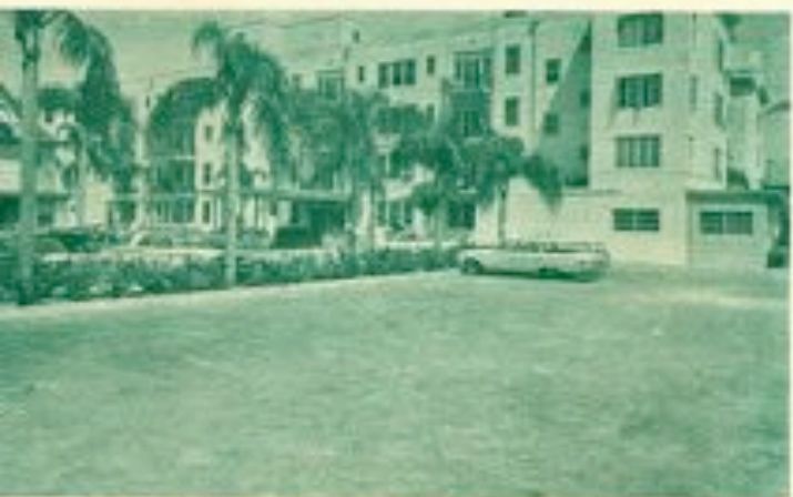
PARKING LOT Plenty of parking space available with lots of room for easy parking.
